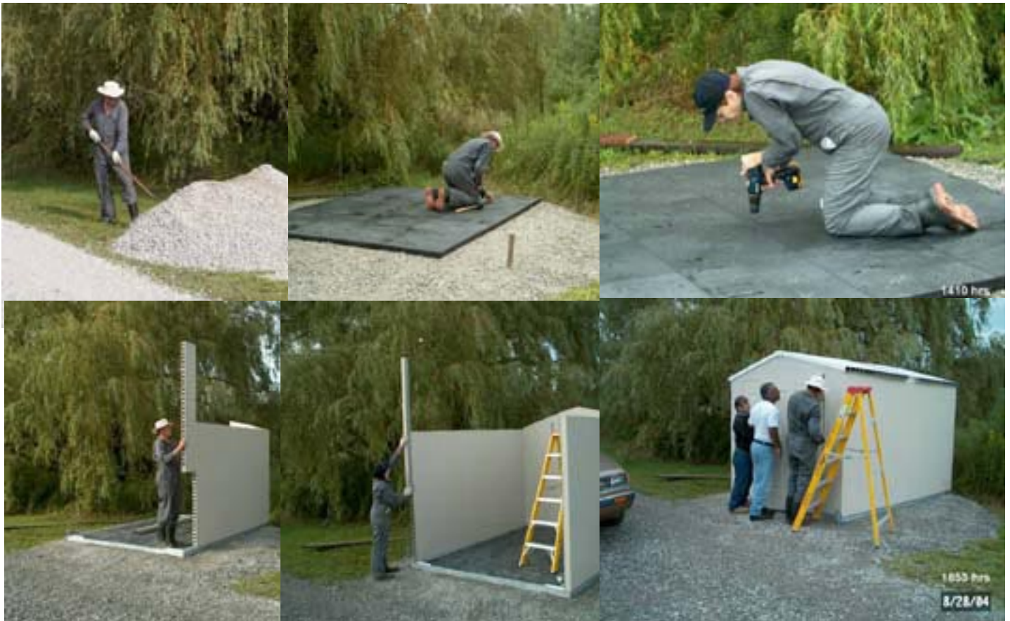
The shed under construction on August 28.
