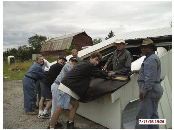
Spring repairs at the CCCA
